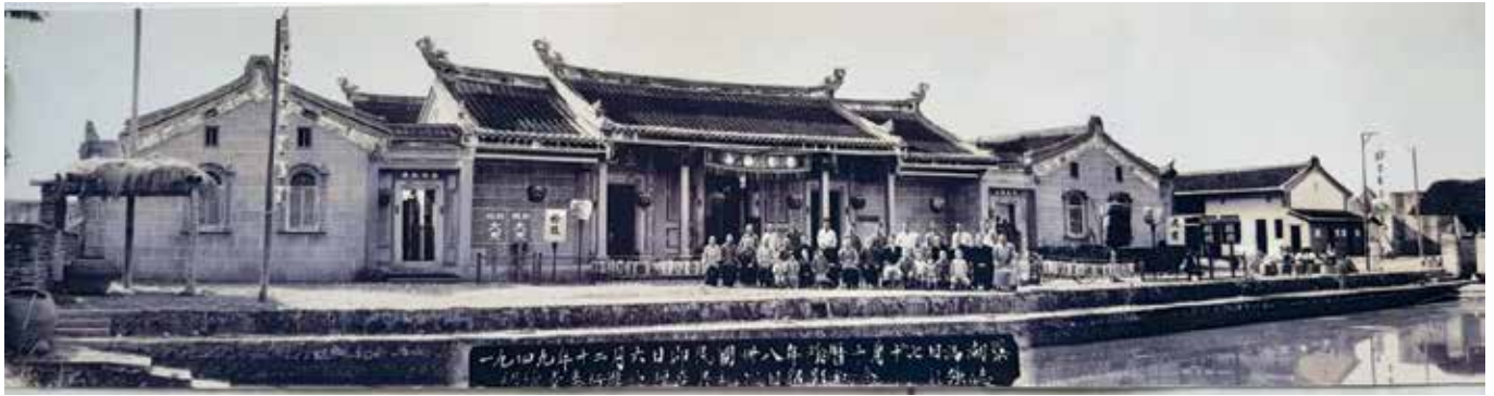
The House that Lam Built. Lam Sen Tong's 100-room mansion in Dabu County.
